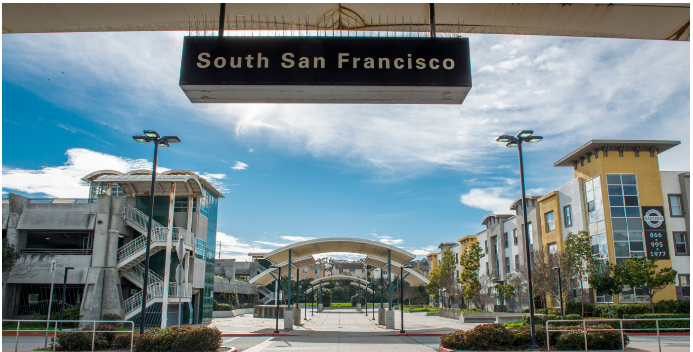
South San Francisco BART Station
