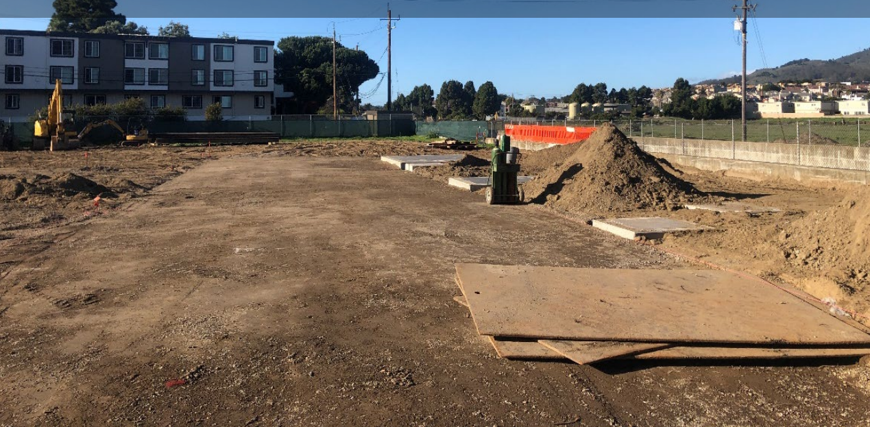
Grit Chamber and Compacted Driveway
