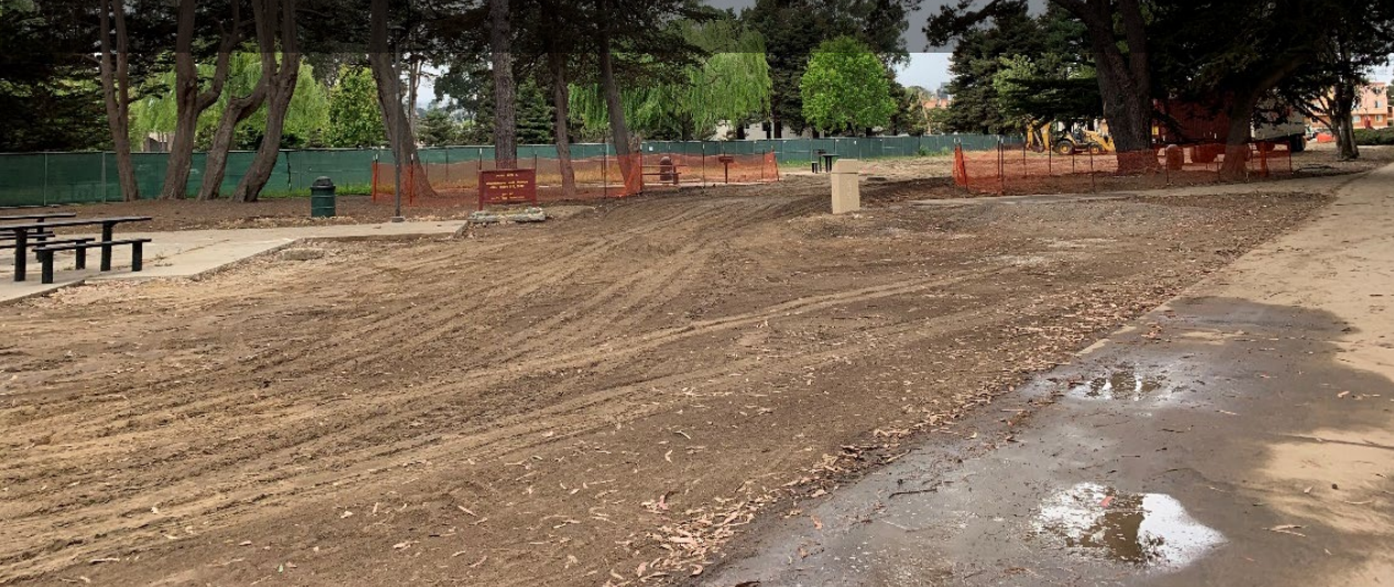
Diversion Pipe Installed Across the Picnic Area
