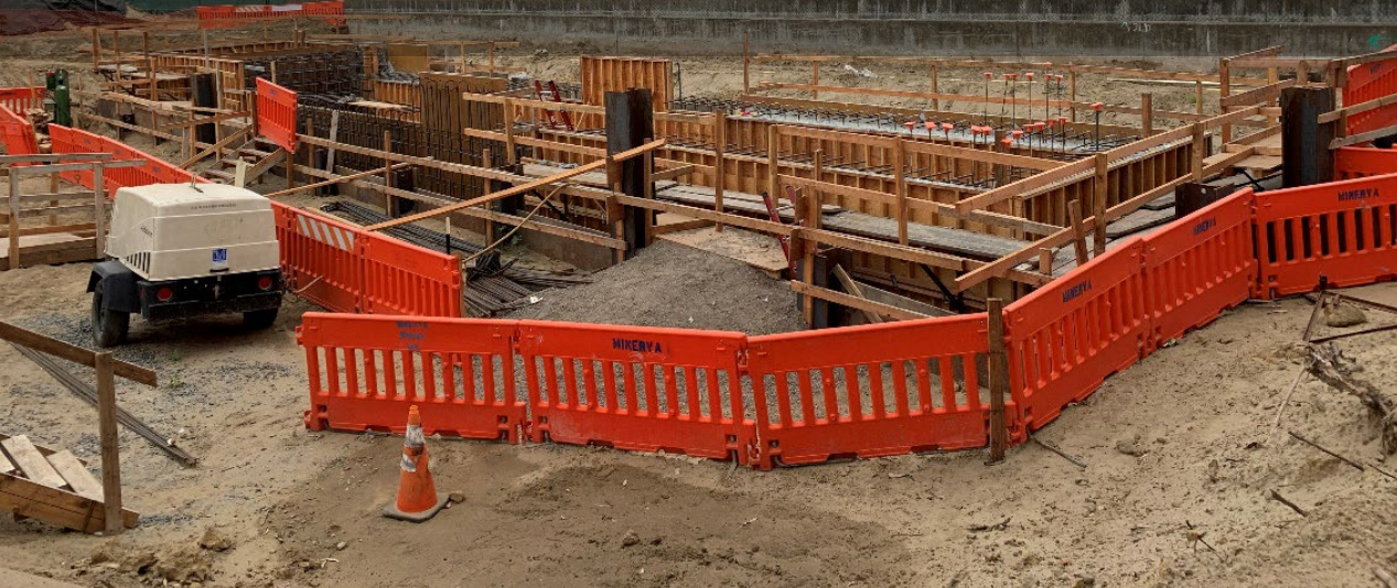
Grit Chamber Structure Wall Concrete Placed
