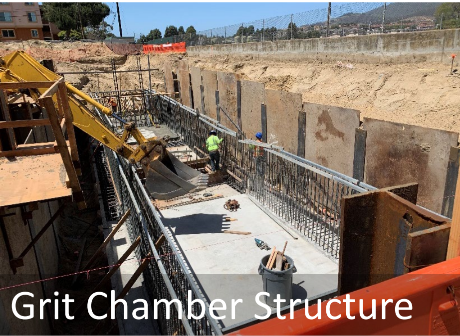
Flow Splitter excavation with slab reinforcing and formwork
