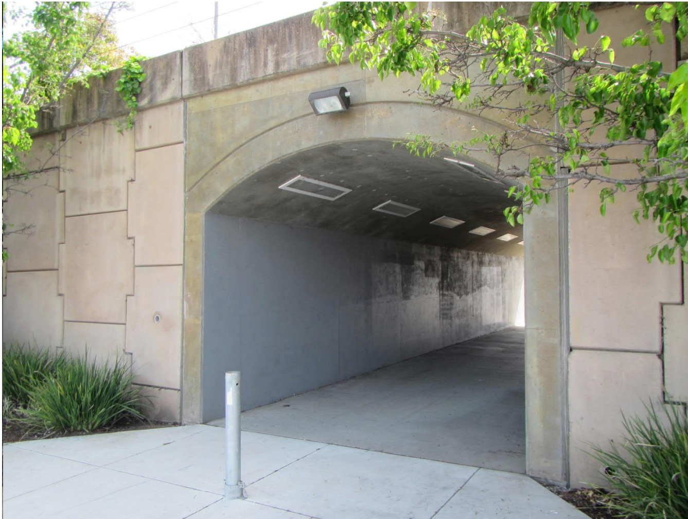
Arroyo Avenue, San Carlos
