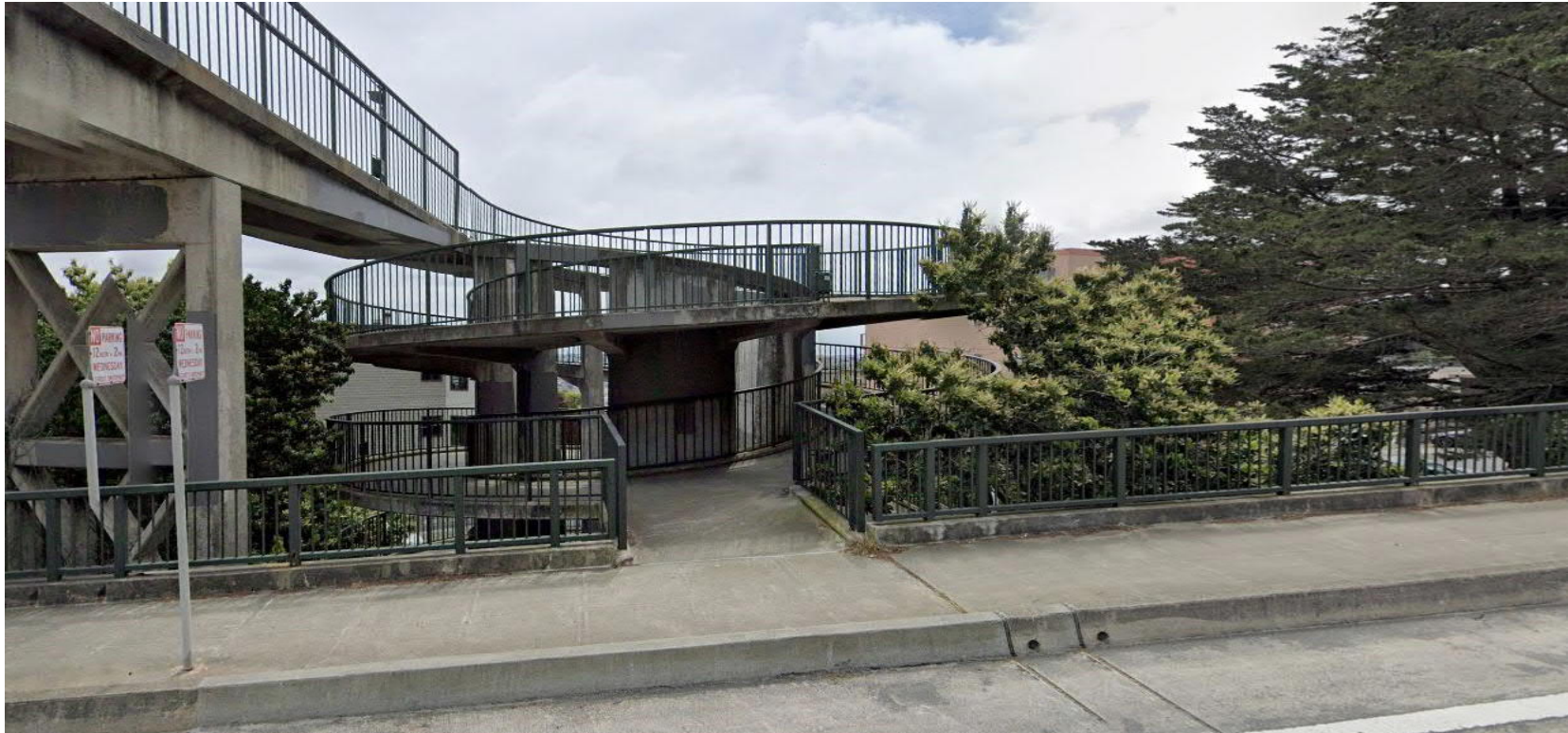
Market Street Overpass, San Francisco
