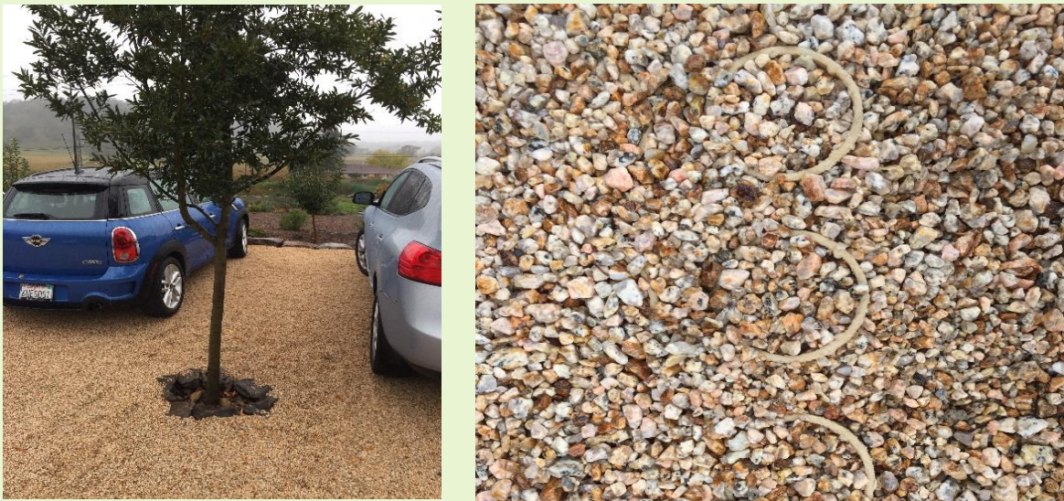
Figure 6-41. Reinforced grid paving in an overflow parking lot in Napa. (Credit: EOA, Inc.)
