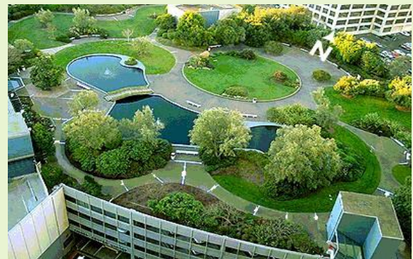
Figure 6-45: Top: Extensive Green Roof at YouTube Headquarters, San Bruno (Courtesy of William McDonough & Partners); Bottom: Intensive Green Roof, Kaiser Center Parking Garage, Oakland. (Credit: Gene Anderson)
