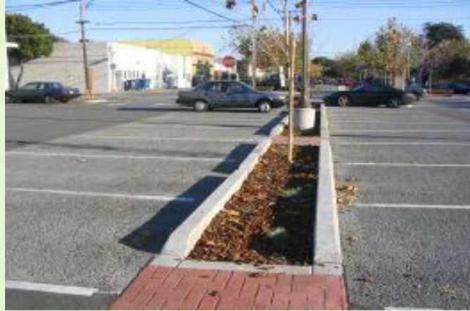
Figure 6-34: The City of Menlo Park used pervious concrete for parking stalls and standard paving in the drive aisles in this public parking lot. (Credit: City of Menlo Park)
