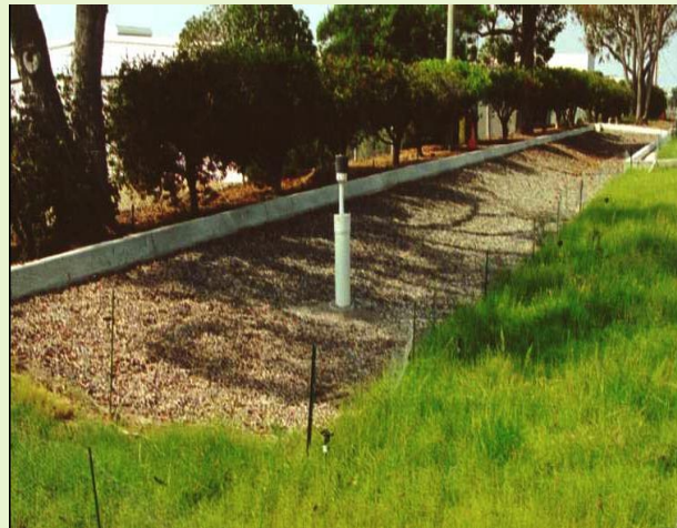
Figure 6-27. Infiltration Trench (Source: CASQA, 2003)
