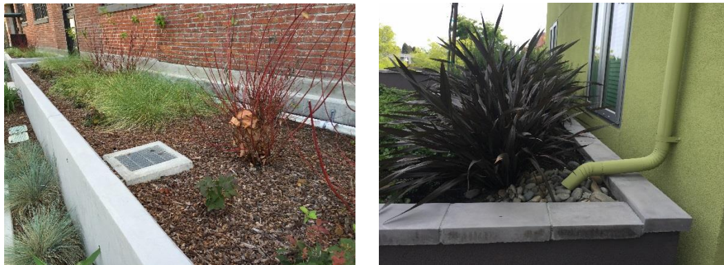
Figure B-4: Typical Flow-Through Planters on-grade (left) and on podium level (right)
