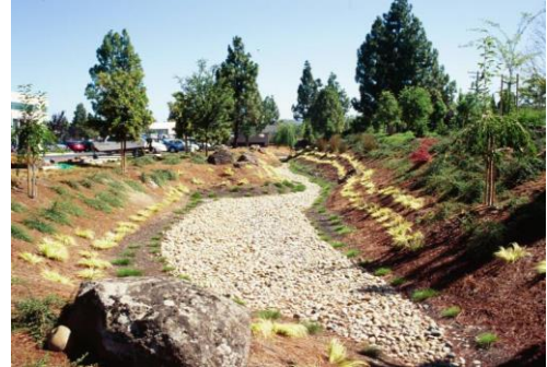
Figure 8-8: Extended Detention Basin, Palo Alto
