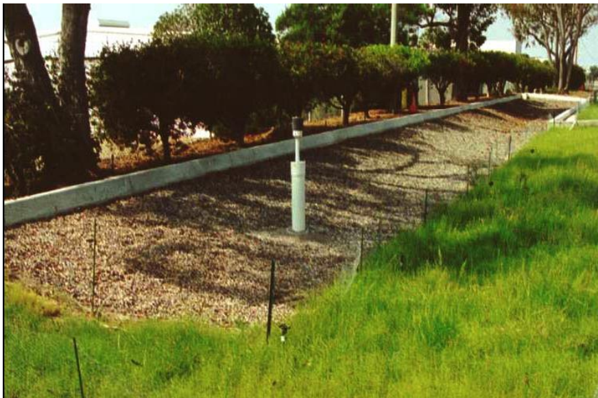
Figure 8-7: Infiltration Trench (Credit: CASQA)
