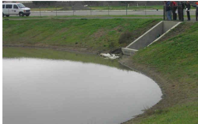
Figure 5-6: Detention pond used for hydromodification management.
