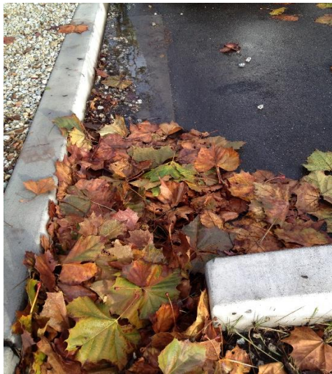
Figure 5-27. London plane tree leaves blocking an inlet (Credit: EOA, Inc.)
