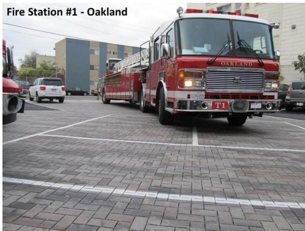
Figure 4-6: Installation of permeable interlocking concrete pavers in Oakland. Water infiltrates through gravel in the joints between the pavers. (Courtesy of the City of Oakland)
