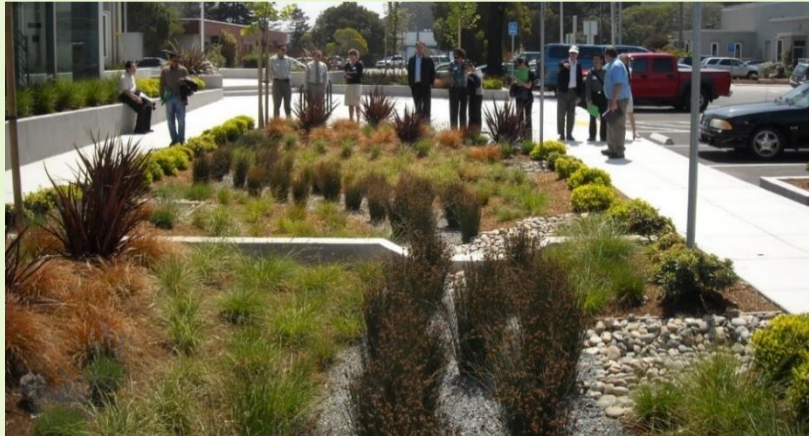
Figure 6-2: Bioretention area (Credit: City of Brisbane)
