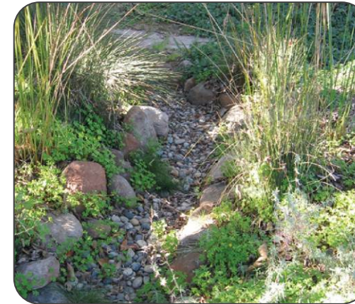
Dry creek infiltrates and conveys runoff.
