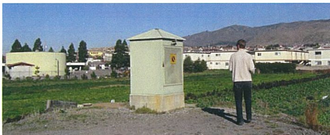
Calwater water wells that require relocation
