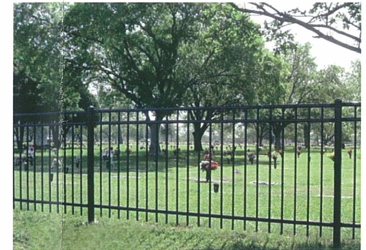
Drainage Channel Fence
