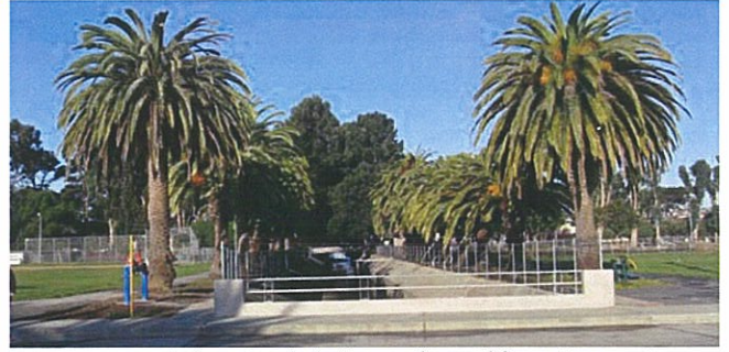
Colma Creek drainage channel from Orange Avenue
