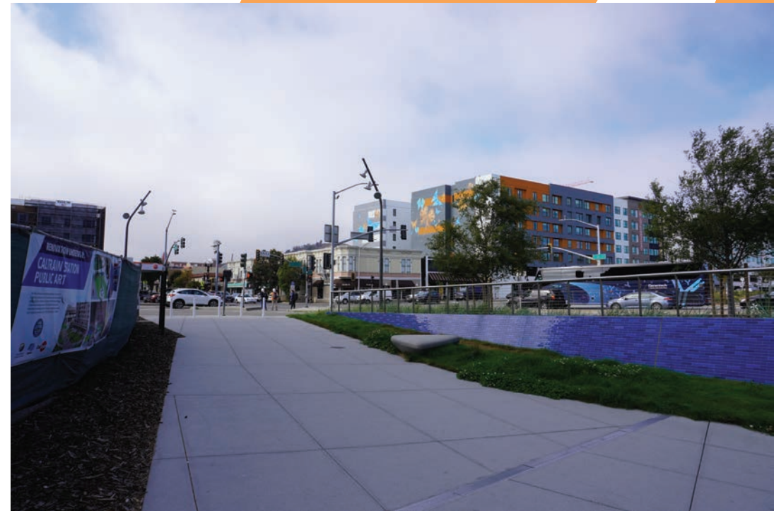
Image: Newly renovated South San Francisco Caltrain Station (2022).
