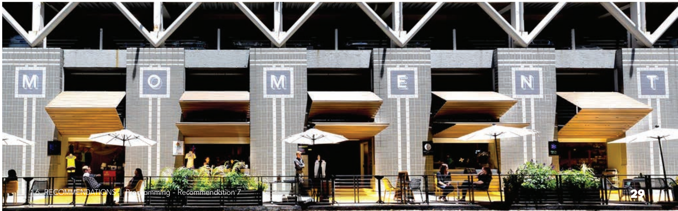
Image: This image shows “Moment San Jose,” a micro retail storefront underneath a parking structure in San Jose, CA.
