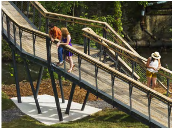
Pedestrian Bridge - Type 1
