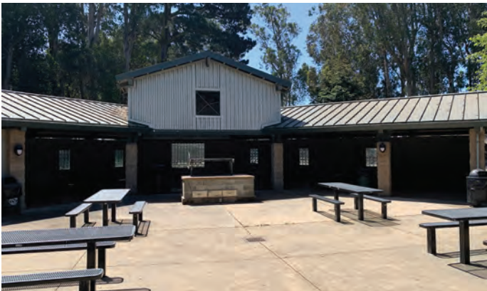
Site Photo - Picnic shelter
