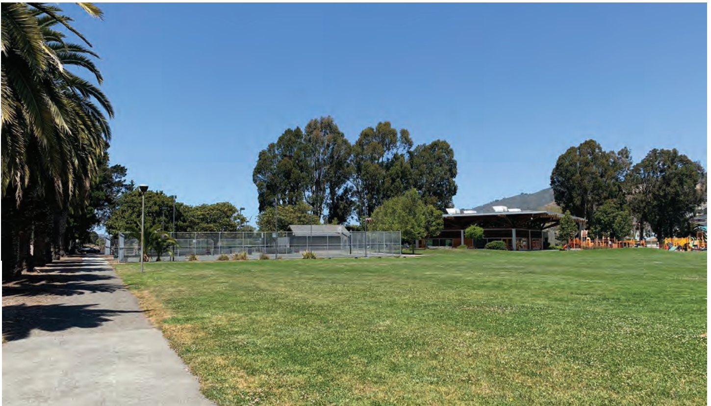
Site Photo - Existing basketball courts and recreation building
