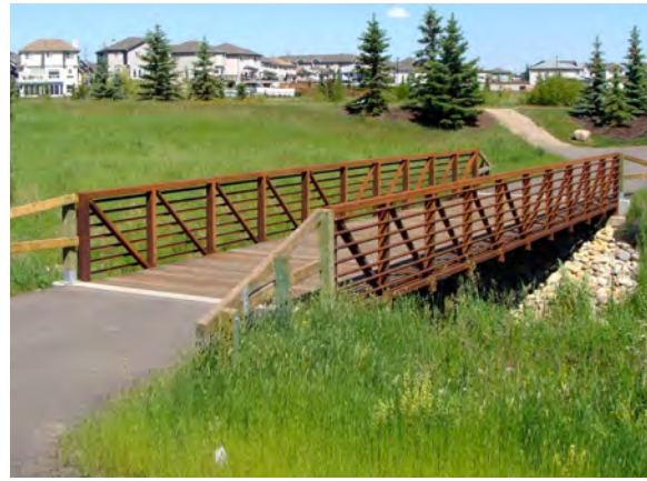
Pedestrian Bridge - Type 2
