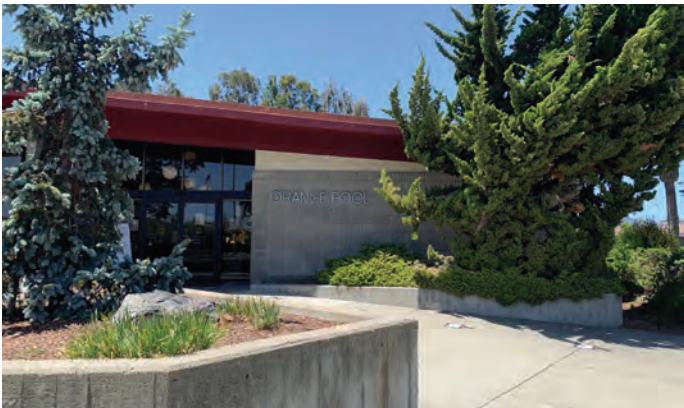
Site Photo - Pool building
