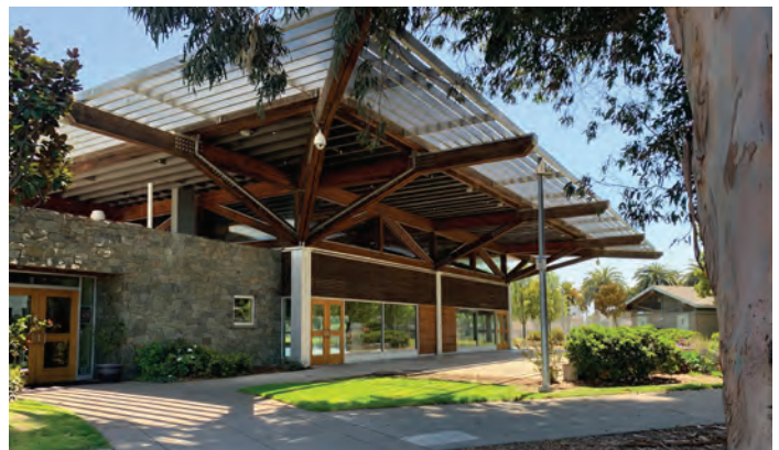
Site Photo - Recreation building
