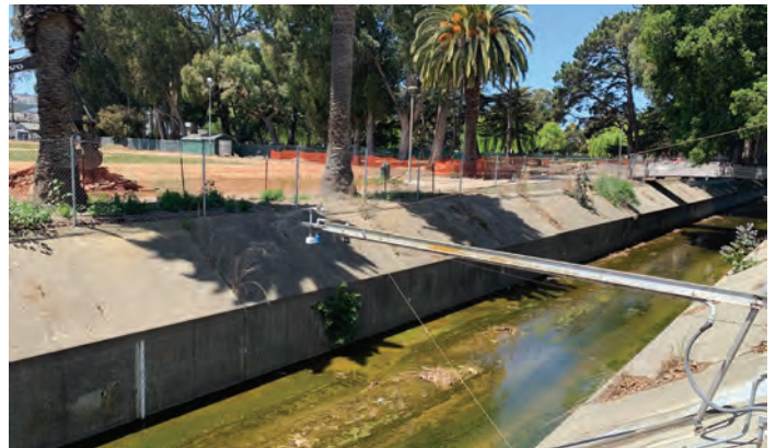
Site Photo - Colma Creek drainage channel
