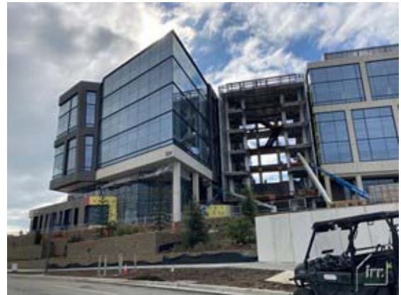
Phase I – Building A & Outdoor Meeting Space
