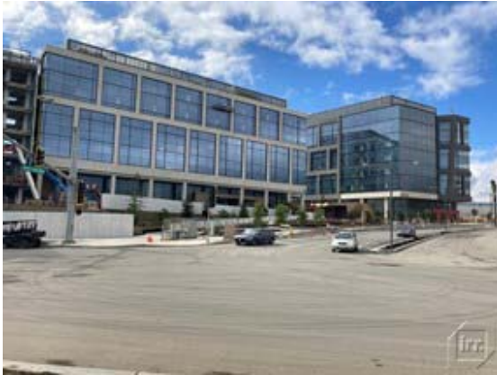
Phase I – Buildings B & C
