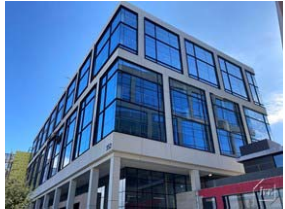
Phase I – Building B
