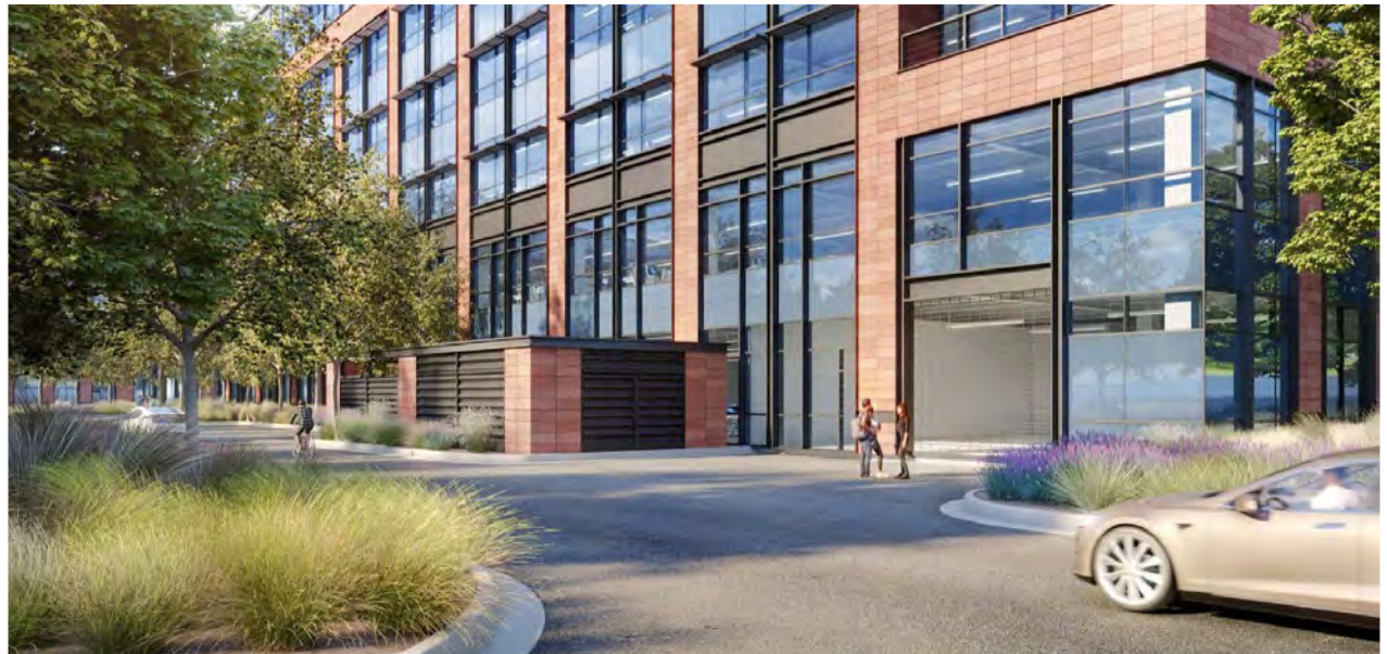
Building 7 - Service Yard
