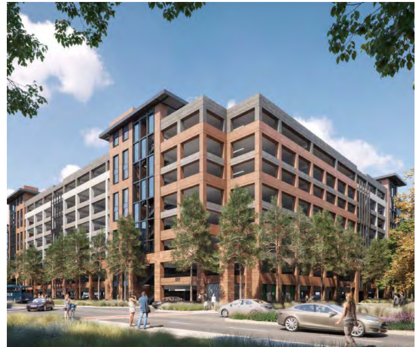
Parking Structure C
