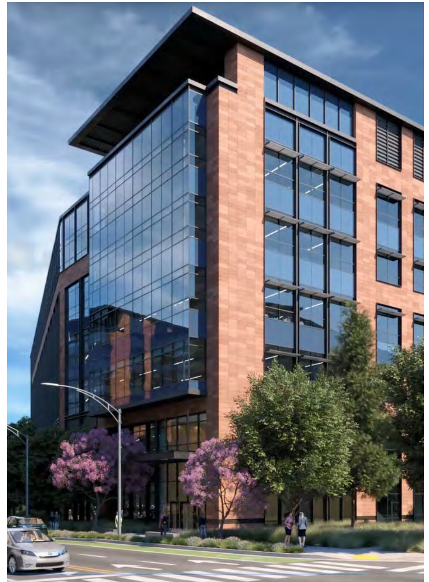
Building 1 - Southeast View
