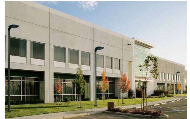
Pole Fixtures Associated with Parking and Roadways
