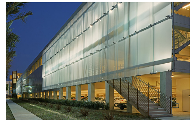
Parking and Service Facades
