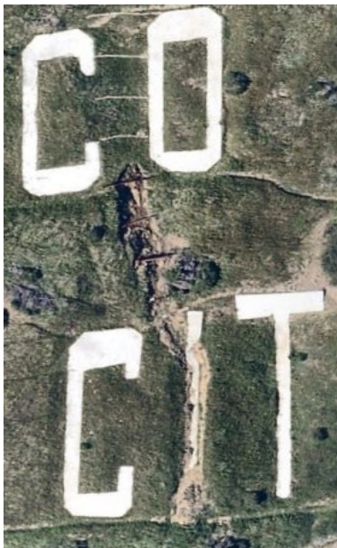
Landslide scar from 2023 storms.
