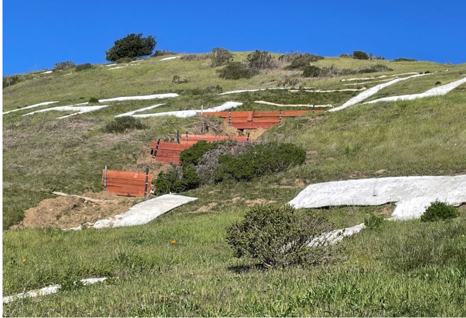
Emergency check dams to control storm erosion between letters.
