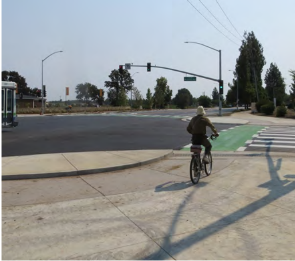
Protected intersections feature a corner safety island and intersection crossing markings.
