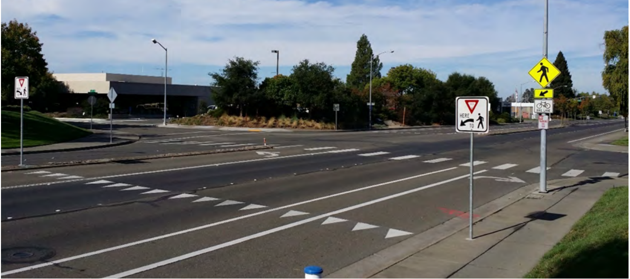
Marked crosswalks at Stony Point Road and Stony Circle
