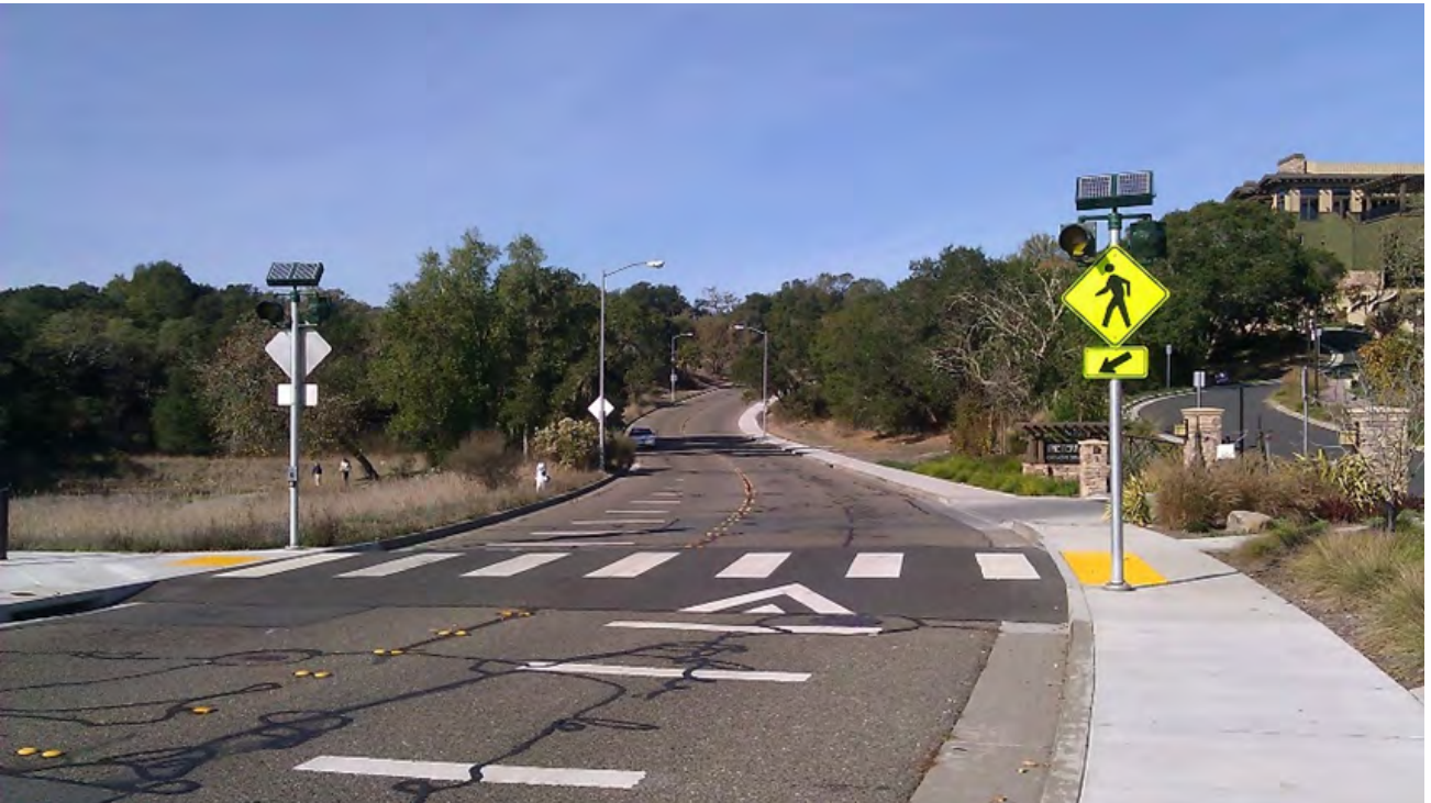
Raised pedestrian crossing on Thomas Lake Harris Drive
