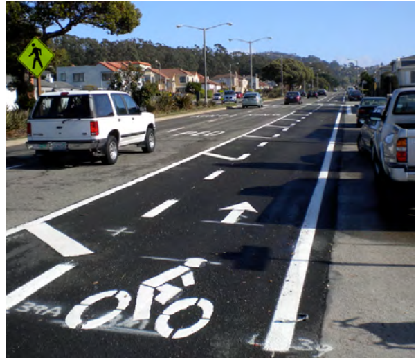
The use of pavement markings delineates space for cyclists to ride in a comfortable facility.
